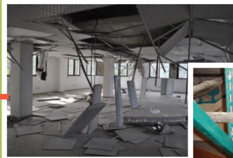
CHUTE D'ÉLÉMENTS D'ÉCLAIRAGE ET PRINCIPE DE FIXATION (©AYHAN IRFANOGLU) (©MARYANN PHOPPS)
