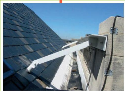
FIXATION D'UN PARAPET (©DEGENKOLB ENGINEERS)
