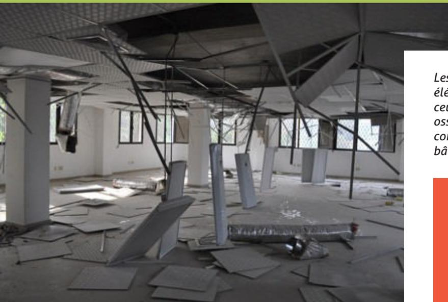
CHUTE D'ELEMENTS NON STRUCTURAUX : ELEMENTS D'ÉCLAIRAGE ET FAUX PLAFOND (©AYHAN IRFANOGLU)
